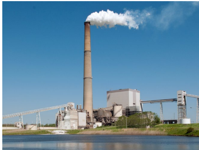
Figure 1: Duke Energy's East Bend Station 600-MWe coal-fired power plant.
