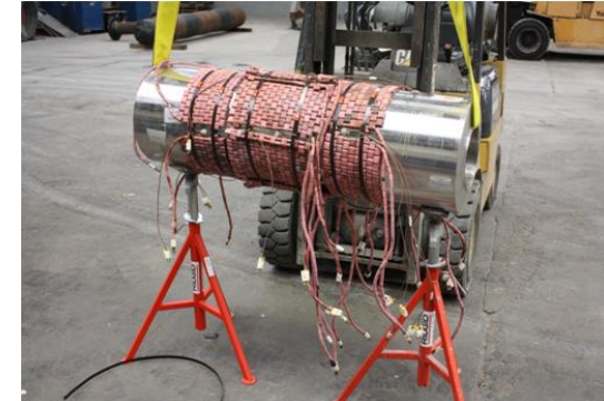
Weld in 3" 740H pipe showing ceramic heating elements used for PWHT
