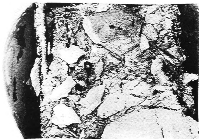
Figure 7. Wet ESP Rod Deck Pluggage
