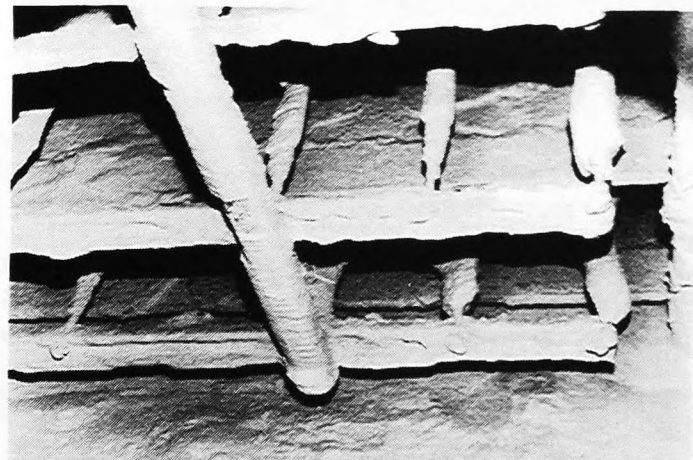
Figure 9. Ash Buildup on Discharge Electrodes in the Dry ESP During LMF5-F
