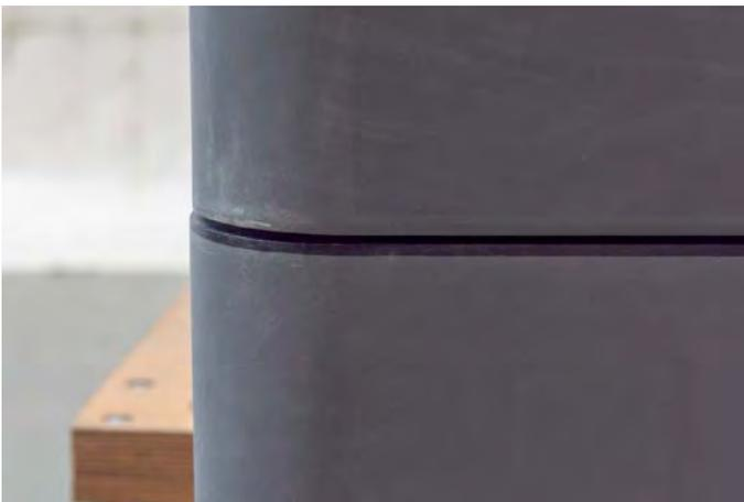
**Figure 3: Four column semi: gap between column and pontoon**
