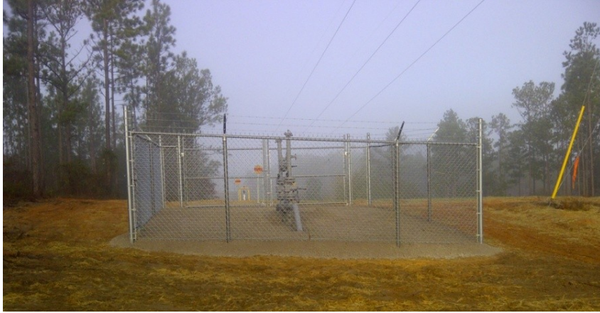
Mainline valve station along pipeline
