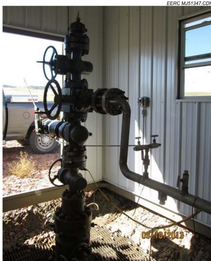
Figure 16. CO 2 or water injector wellhead (taken from Rawson, 2014).
