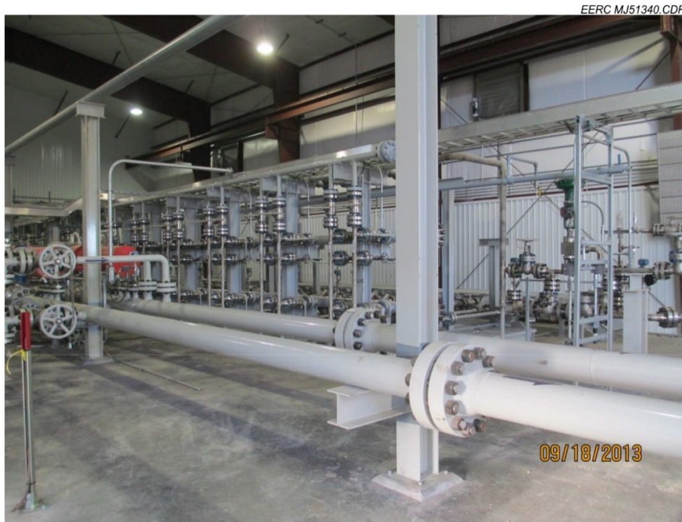
Figure 9. The Bell Creek test site production manifold (taken from Rawson, 2014).
