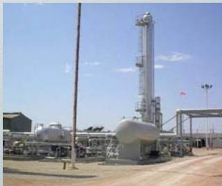
An Amine Capture Plant on a Gas Processing Plant Photo provided by CONSOL Energy
