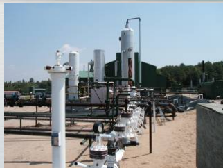
Active CO 2 EOR Flood with several additional wells present
