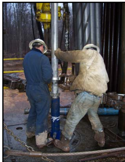
Figure 5. Drilling the Test Well
