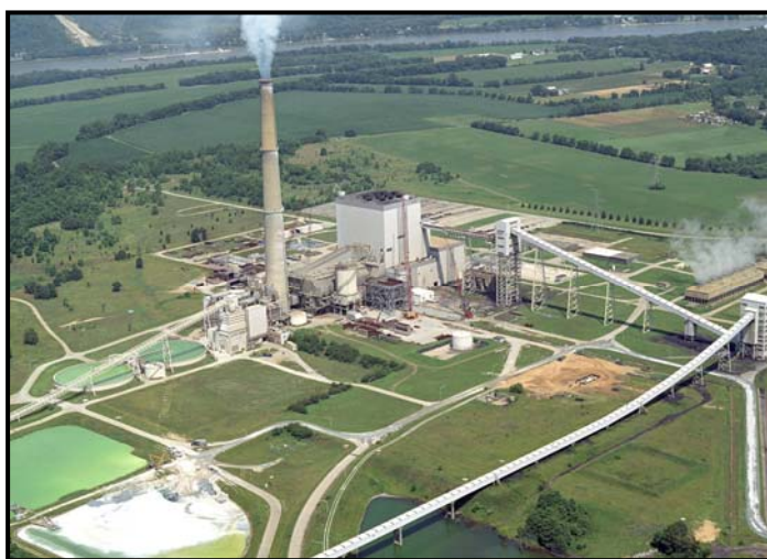
Figure 1. East Bend Generating Station
