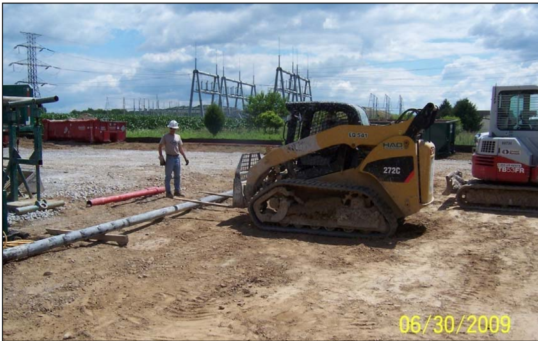
Figure 3-9. Photograph of the Core Barrel after Collecting the Second Core
