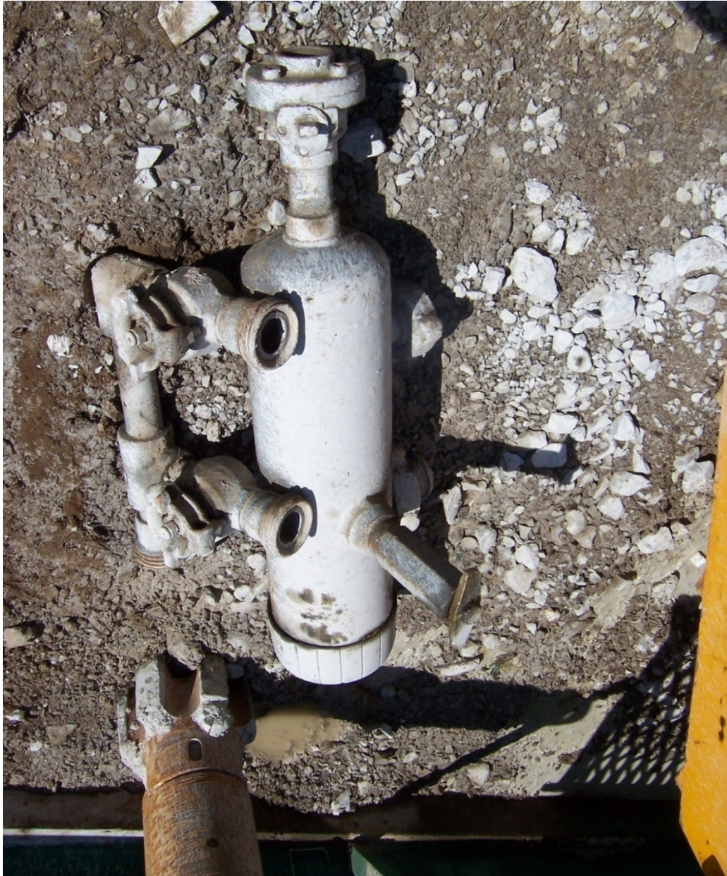
Figure 3-8. Photograph of Cement Head Used on the East Bend Well
