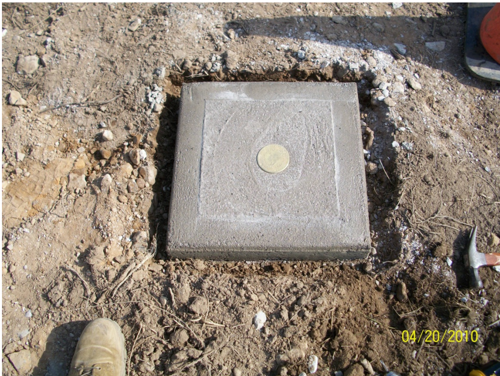
Figure 9-2b. Concrete Marker Emplaced Above Well, Including Brass Tag with UIC Permit Number and Other Identifying Information
